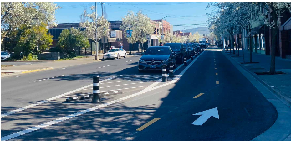
Two-way bicycle facility on Main Street in Downtown Medford.
