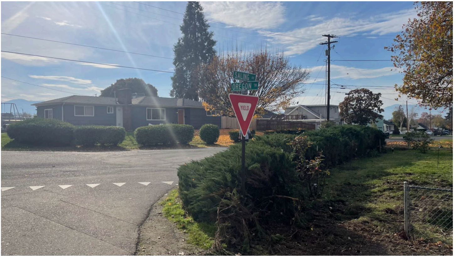
Photo 5: Limited visibility for right-hand turn from Oregon Terrace onto Saling.
